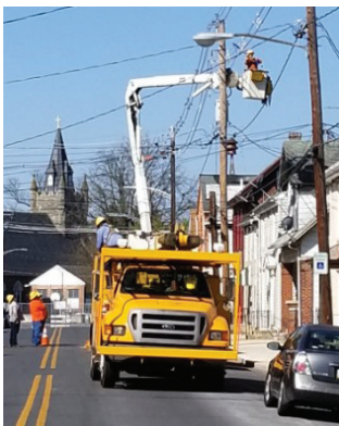
Working on Feeder Tie Along Broad Street
