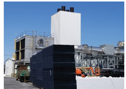
Orchard Park Generating Station Cooling Tower Rebuilds
