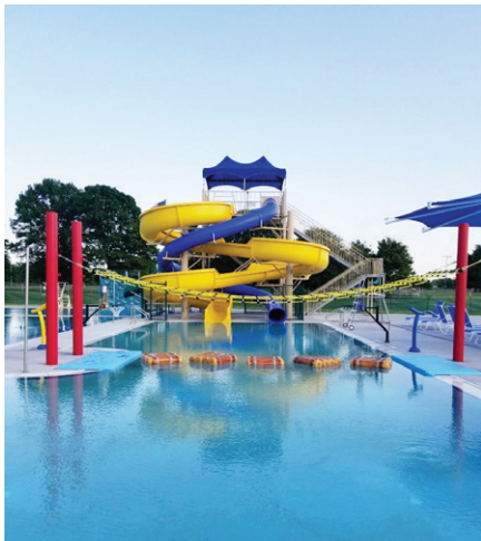
Chambersburg Aquatic Center
