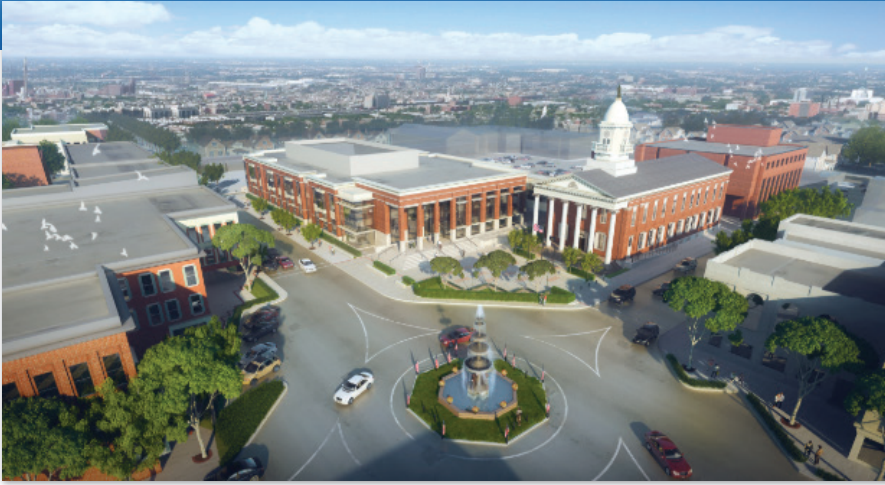
In 2019, Franklin County is expected to begin construction of a new Twenty-First Century Judicial Center on Memorial Square in Downtown Chambersburg
