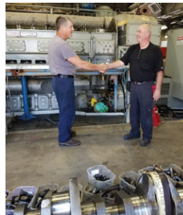
Falling Spring Generating Station #7 Rebuild
